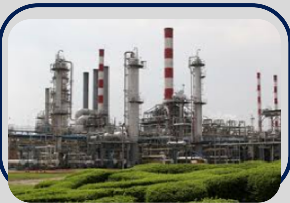
1. Oil & Gas Plant
